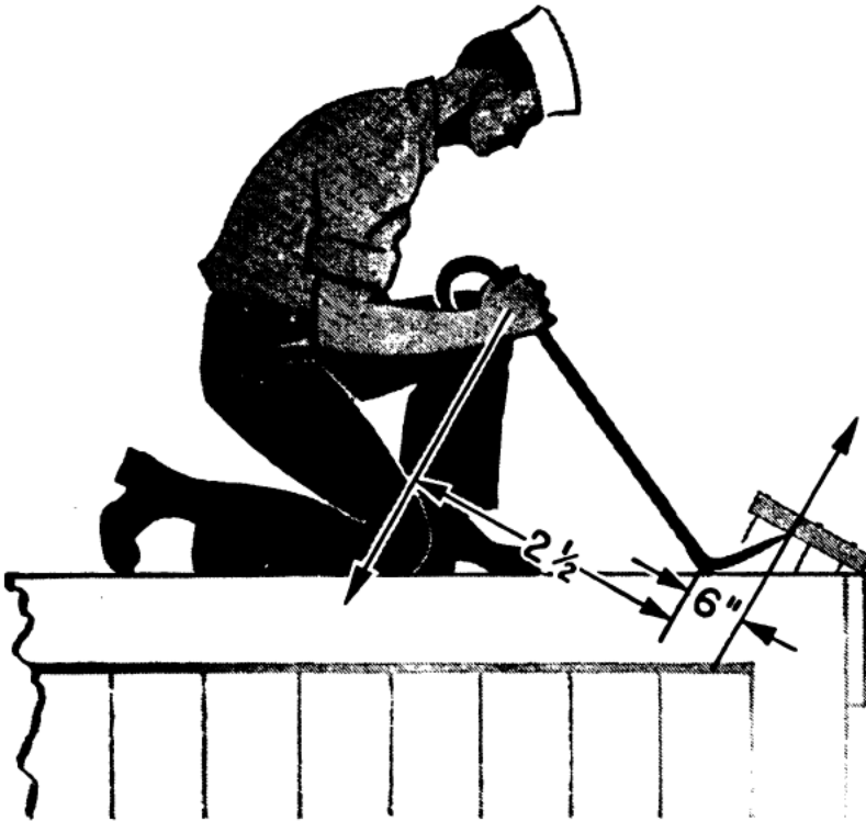
Figure 11.—Using a wrecking bar.
